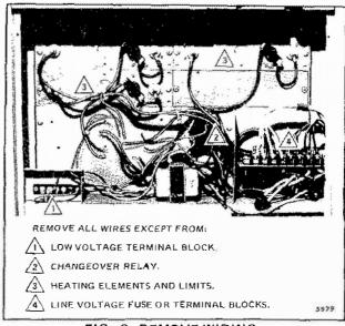
FIG. 3-REMOVE WIRING.
