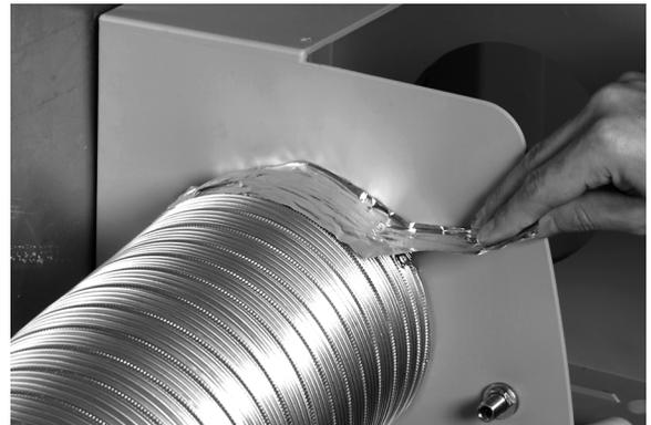
**Fig. 15. Sealing connections with tape.**
