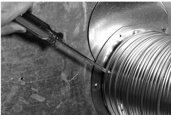
**Fig. 13. Connecting Bypass Duct to Bypass Collar.**
